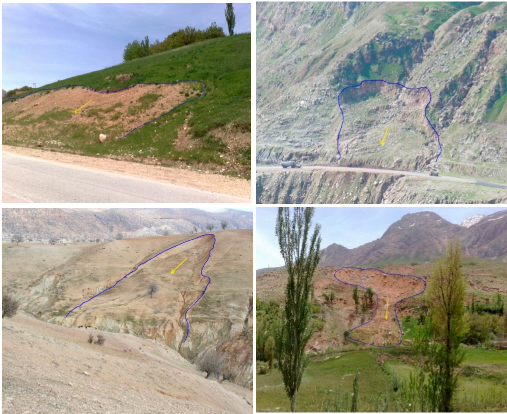
Figure 2. Some recent landslides in the Sarkhoon watershed.
