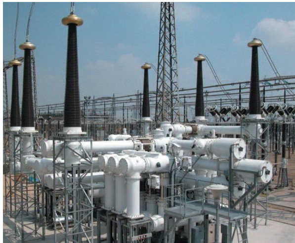
3DQ1 switchgear for rated voltage 420 kV
