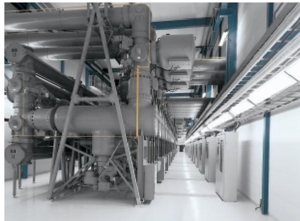
3DQ1 switchgear for rated voltage 420 kV
