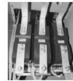
Cable and CT compartment
