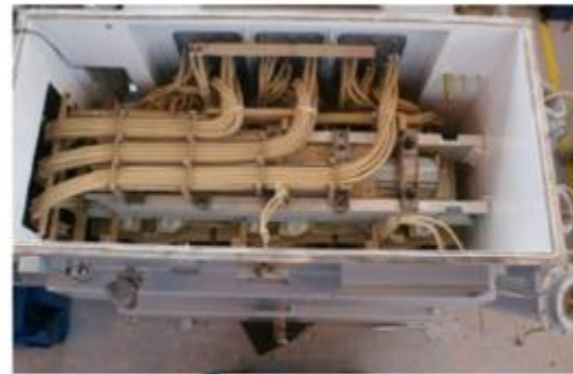
Tanking: ratio, core-to-ground, in-tank C/B - polarity, ratio, saturation
