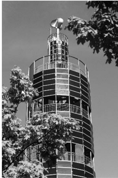
Figure 6.15 Solar Tower, Training and Technology Center Handwerkskammer Heilbronn, Germany. Wuerth Solar frameless CIS Façade modules with a total nominal power of 8 kW p (STC) were installed in April 2001. The installation comprises 120 modules with the dimensions 60 cm by 120 cm and 40 modules with the dimensions 40 cm by 60 cm. Reproduced with permission of Wurth Solar GmbH & Co.KG.
