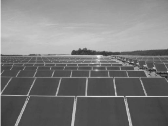
Figure 5.22 World's largest 1 MWp amorphous silicon solar power plant in the German city of Bittenwiesen in the suburbs of Munich. (With permission from Phonix SonnenStrom AG).
