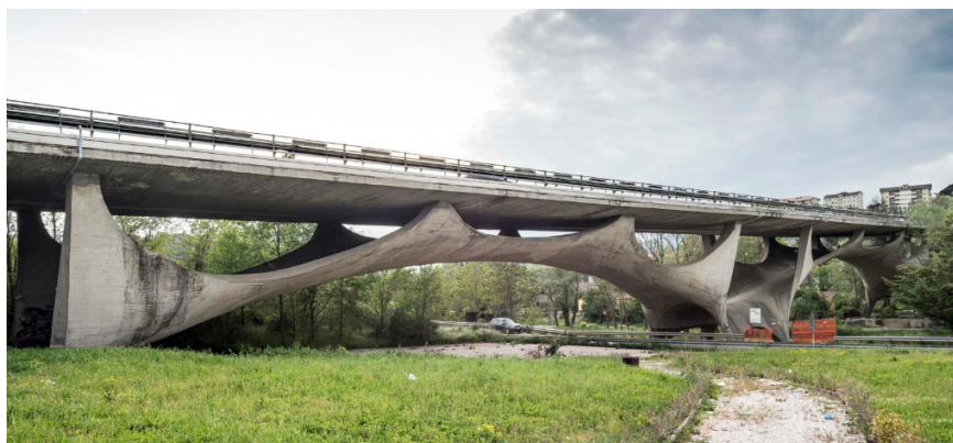
Figure 12. The Musmeci Bridge, Italy (Aloarchitettiroma, n.d.)
