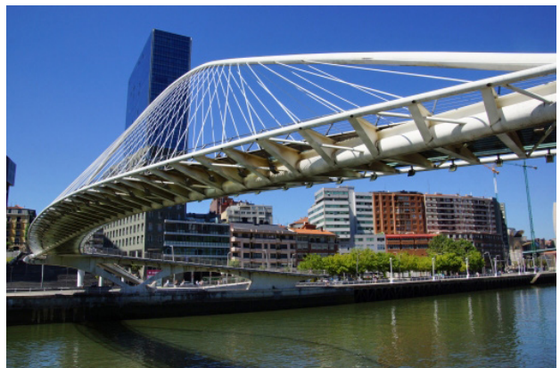
Figure 3. Campo Volantín footbridge, Spain; mechanical mimicry of the spine (Structurae, n.d.)
